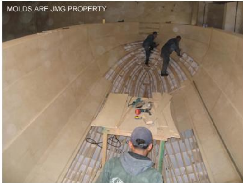
PILOT BOAT 12 MOLD CONSTRUCTION HULL
